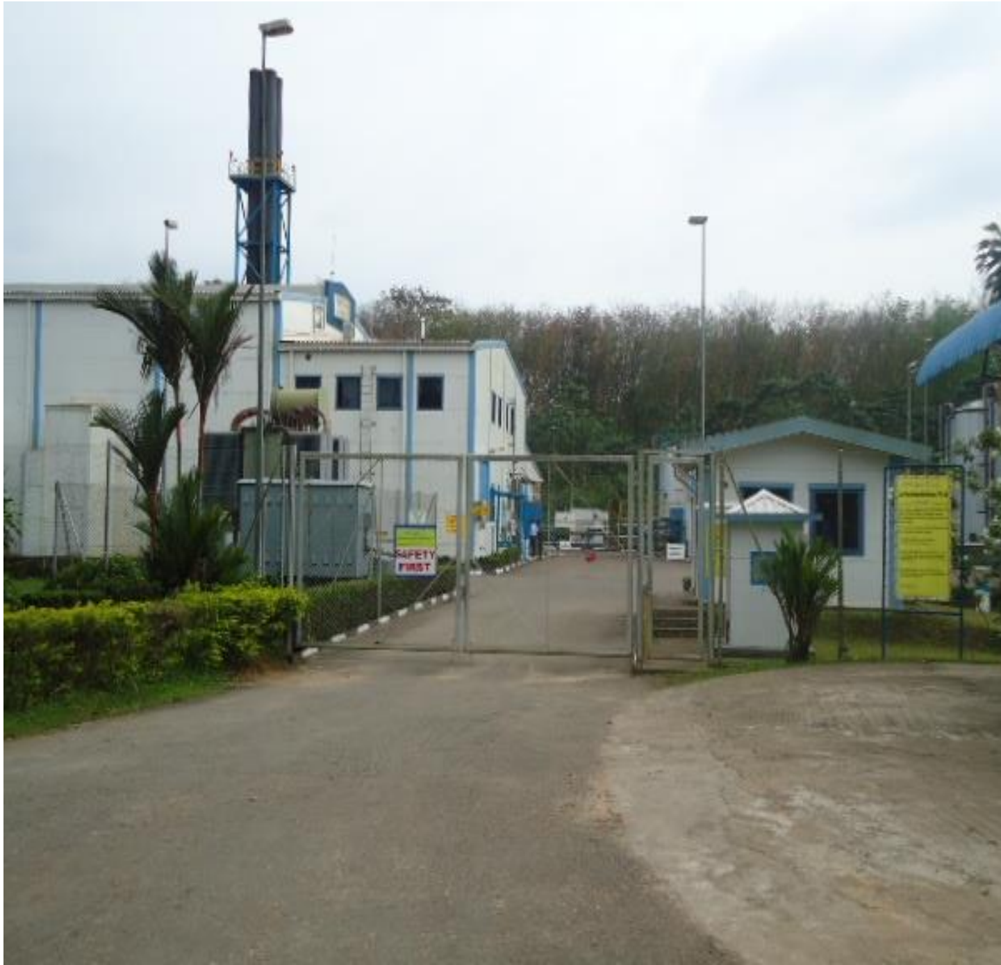
Figure 1 - Plant Main Entrance
