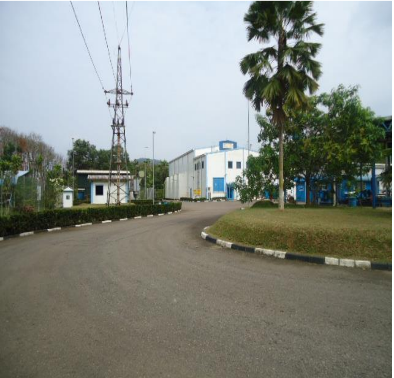
Figure 3 - Plant Access Road
