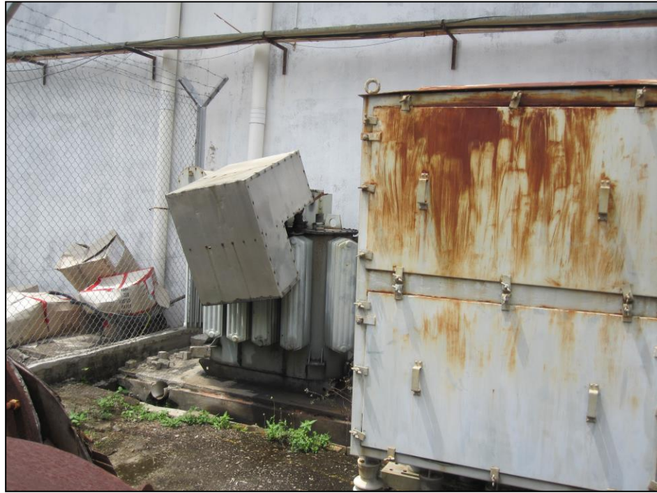
Photo of Transformer
