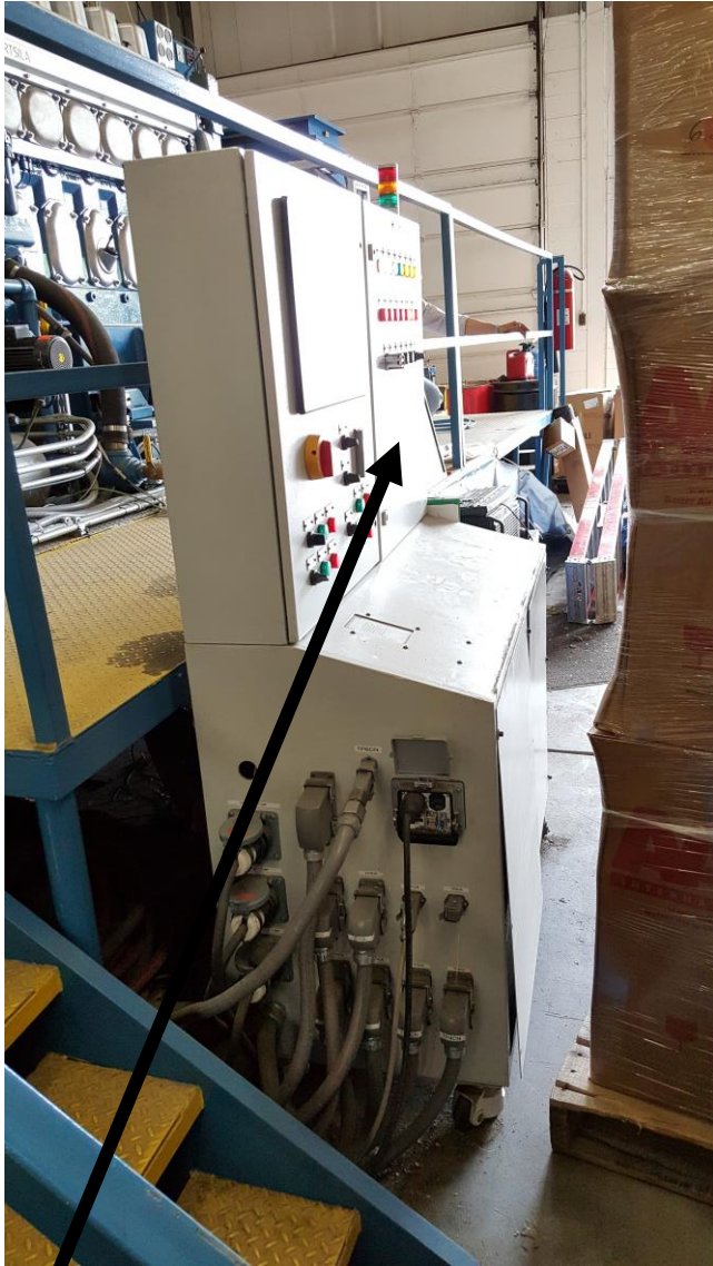
#3 Start/Stop System (Control Panel)
